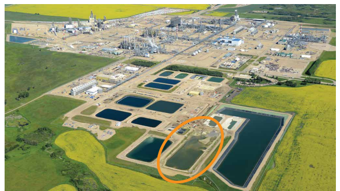
Aerial of Joffre Site highlighting the location of the existing southeast retention pond that will be remediated.
